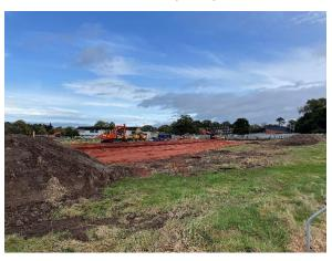
Wolverhampton College's land, the foundations are being dug, readying the site for the services to be connected to the B-block of our existing buildings. A service trench will be dug in sections across the site to connect the two structures with electricity, water and a high-speed internet connection. We will notify you when this work is taking place. The trench will be protected with barriers to prevent access by
